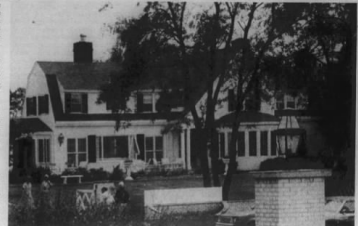
Community of Jesus compound on the shores of Rock Harbor in Orleans includes this traditional clapboard frame house. The non-denominational Christian group wants to build a 104-foot tall stone gothic church near the site.
